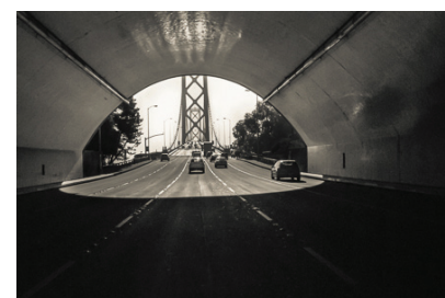
Yerba Buena Tunnel Bay Bridge, San Francisco
